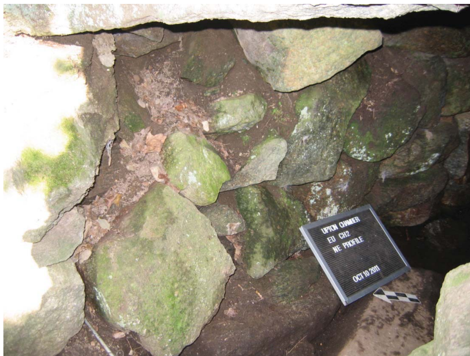
Plate 33. EUs CH1 and CH2 northeast profile of chamber wall, view east; note gaps in stonework where soil is infilling.
