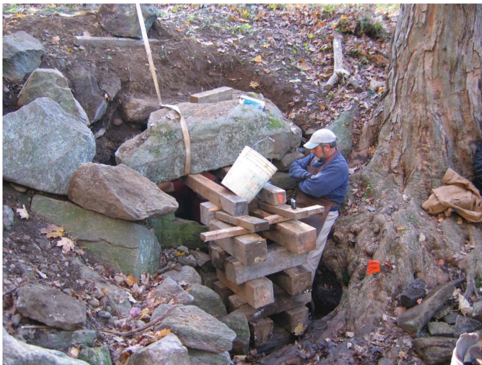
Plate 34. Wood cribbing in place at the Upton chamber entrance with the in-situ lintel further secured with a strap, view south.
