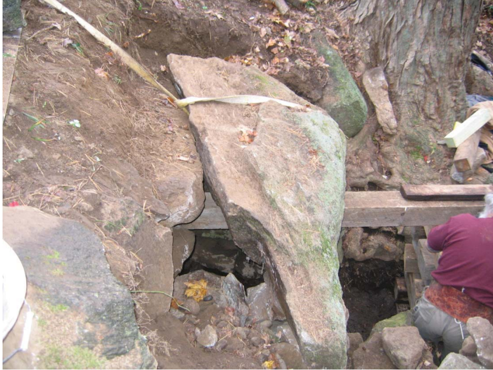
Plate 42. Stonework rehabilitation in progress, lintel shifted back with gap to be closed with re-use of fallen ceiling boulder from EUs CH1 and CH2, view southwest.
