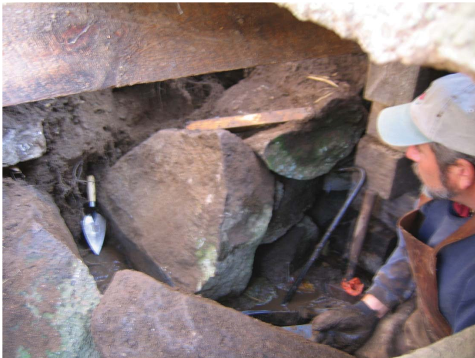
Plate 39. Stonework rehabilitation in progress in the north chamber wall above EU CH1, view east; the trowel is pointing to lowest course of stones in the chamber wall.
