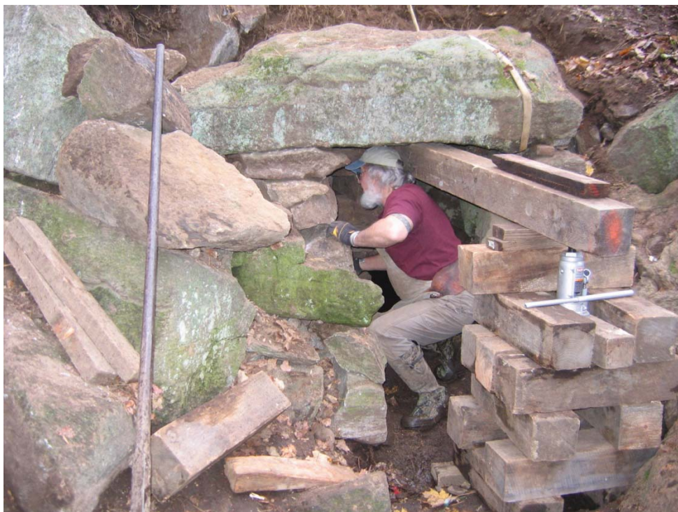
Plate 41. Stonework rehabilitation in progress in the north chamber wall above EU CH1, view southeast.
