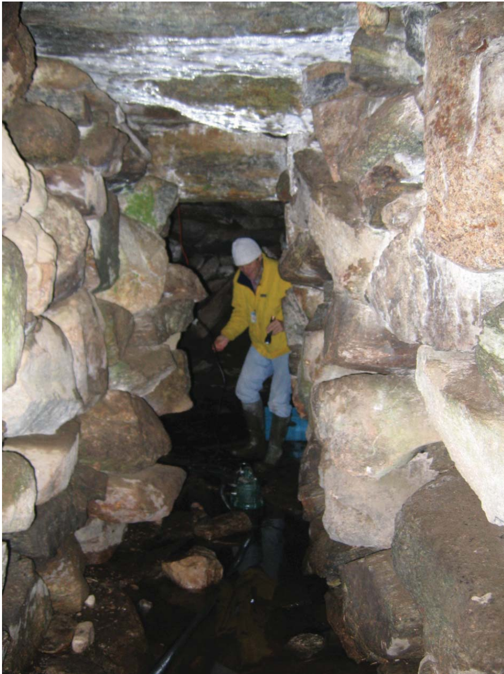
Plate 7. Pumping water from the main chamber; view southeast of flooded chamber passageway from the chamber entrance.
