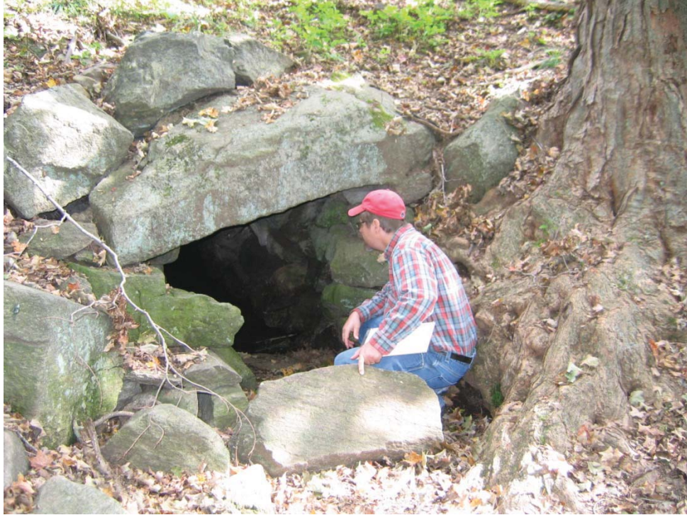
Plate 1. Existing conditions of the Upton Chamber entrance prior to field work, view southeast.
