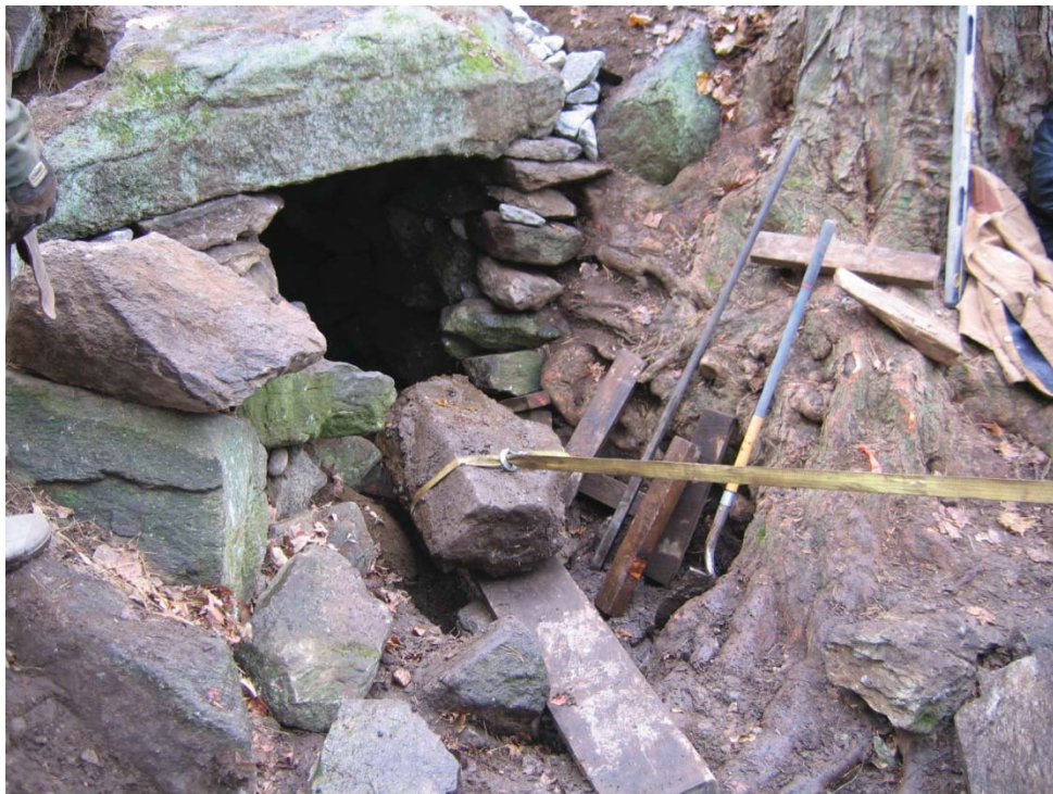
Plate 43. Stonework rehabilitation of chamber entrance completed and cribbing removed; the fallen ceiling boulder from EUs CH1 and CH2 is being winched out for reuse behind the lintel, view southeast.
