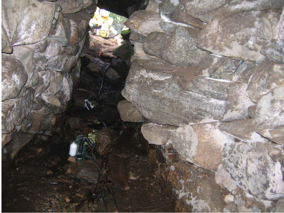
Plate 8. View northwest of chamber passageway from inside the vaulted main chamber after water removal; note debris of wood boards on chamber floor.
