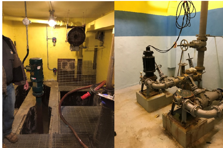
Influent Channel Grinder and Pumps
