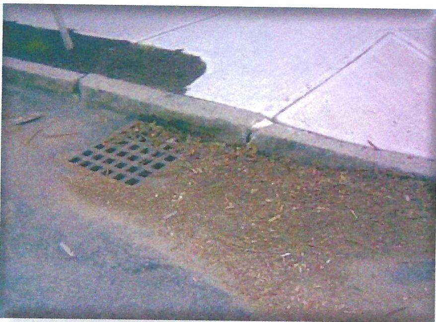
**Description:** Deep sump catch basins, also known as oil and grease or hooded catch basins, are underground retention systems designed to remove trash, debris, and coarse sediment from stormwater runoff, and serve as temporary spill containment devices for floatables such as oils and greases.
